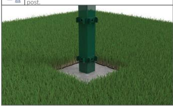
Lift the mesh panels into position between the posts, ready for fixing. Making sure the panel is evenly spaced between posts and the mesh is attach to the 'U' clips on the post.
